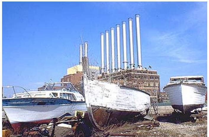
The original Seven Sisters and Two Brothers power plant
